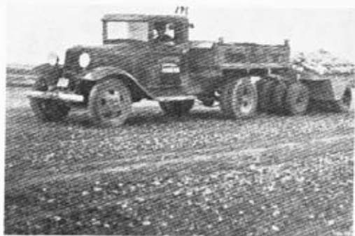
FIG. 4.—Runway Construction at Medicine Hat, Alta., Wobble Wheel Rubber Tyred Roller Compacting Base Course.
