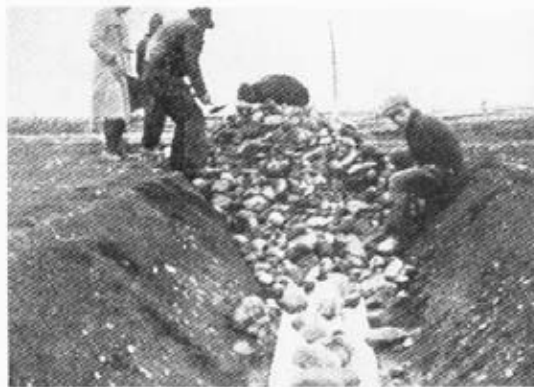
FIG. 8.—Stone Filled "V" Ditch.
