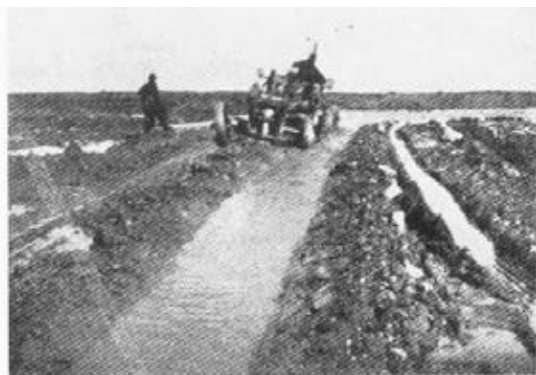
FIG. 7.—Airport Drainage—Using Blade Grader for "V" Ditch.
