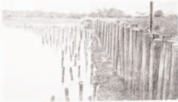
Photo No. 4. Photo taken from southern end of bridge showing initial stage of covestment works and light poles driven in the stream bed.
