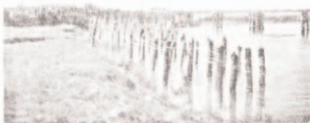
Photo No. 3.—Light poles driven by light pile-driver and connected by plank with designed to slow up the river flow and cause silting
