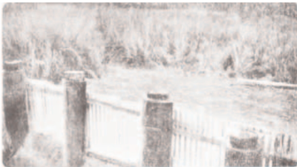
Photo No. 1.—Treatment with poles backed with old rails and galvanized corrugated iron sheeting
