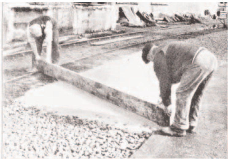
Fig. 5.—Roadwork: Screeding the surface after grouting.
