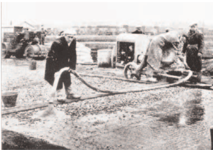
Fig. 3.—Grouting direct from the machine into the stone.
