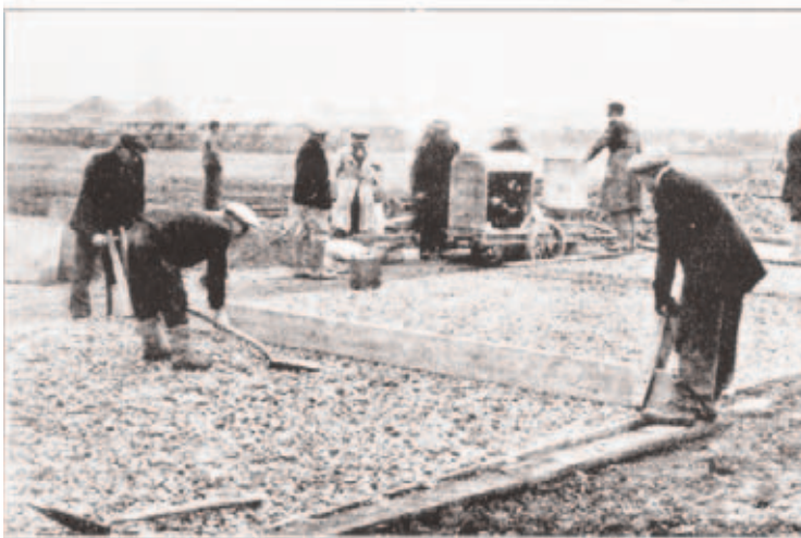
Fig. 4.—Roadwork; levelling the aggregate before grouting.
