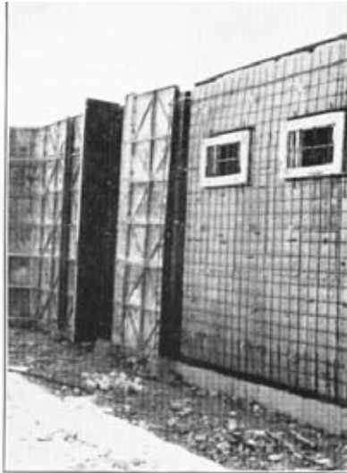
C.—Partially erected shuttering. This shows clearly :— (a) The stiffness of the shuttering. (b) The method of framing in the windows. (c) The reinforcement. (d) The heat insulating material built up against the inner shuttering.
