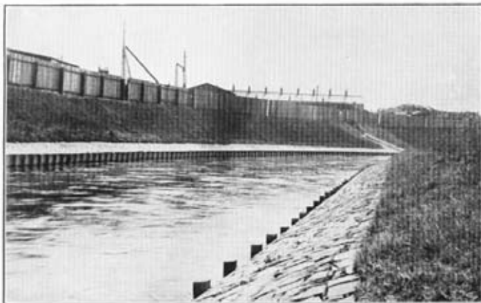
2.—River Mersey. Showing completed piling (steel and timber) and bank toe revetment.
