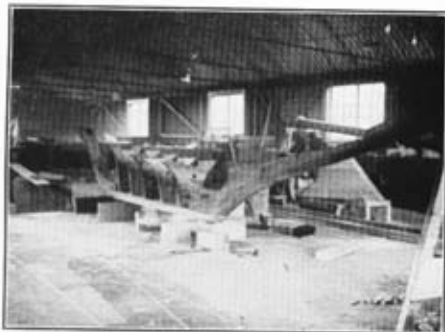
1.—(Nov., 1937.) The backbone set up. Note the deadwood and strainer in rear, and the oak floors.
