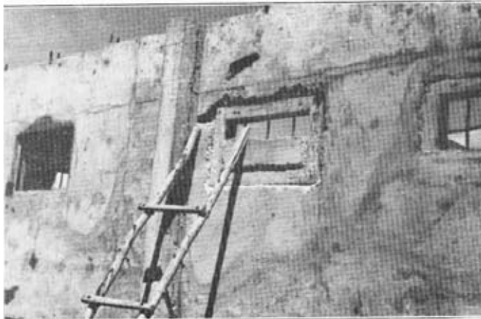
F.—A leak in the framing round a window. Result:—A partly solid window and a bad hole above it.
