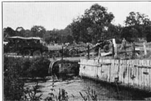
4.—Gun on bridge at D. Dragon on S.B.G. at E. Note unorthodox use of S.B.G. launching hoses, as wheel guides!
