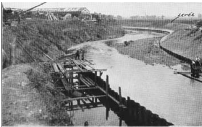
3.—River Mersey. Driving interlocking sheet steel piling.
