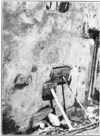
H.—Patching. Bad honeycomb places, as in G, cut out and patched.
