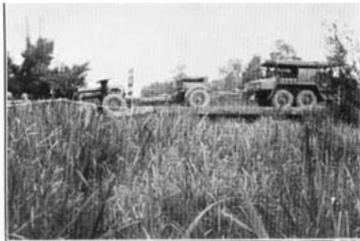
2.—Completed bridge at B. The first crossing, heavy bridge on R.S.J.'s over total 63 ft.
