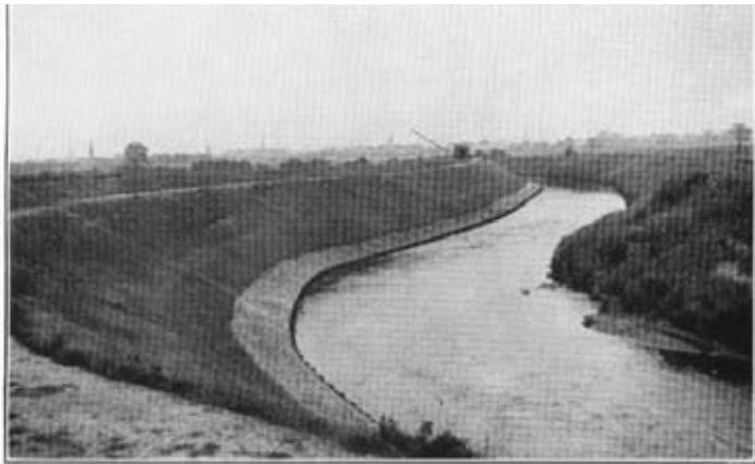
1.—Toe revetment and flood bank.
