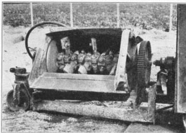
Fig. 1.—A 3-cu. ft. single-shaft mixer for stabilized soil.
