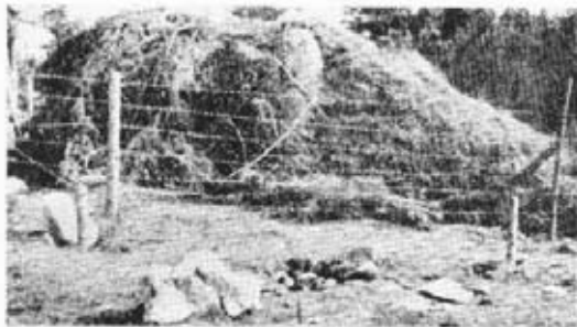
PHOTO No. 7.—Completed and camouflaged medium post. The enemy side is on the right. The M.G. loophole is visible, also the upper portion of the protecting buttress "ear."
