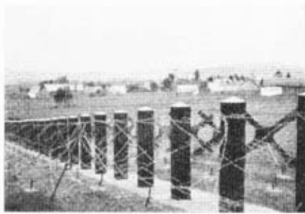
Photo No. 16.—Each column is made up out of two upright iron channels, standing in a concrete socket. The uprights are welded together and then filled with concrete.
