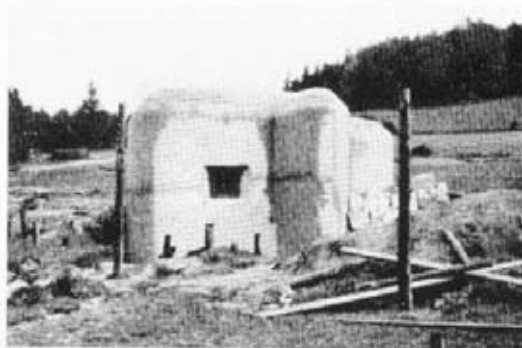
PHOTO NO. 5.—Incomplete medium loopholed post. The enemy side is on the right. A machine-gun loophole is visible, protected on the front by a projecting "ear." The layer of protective stone is in course of construction. This so-called "detonating layer" is designed to catch dropping shells or mines, which it deflects and causes to explode prematurely before they reach the reinforced concrete wall.
