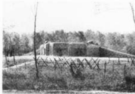
PHOTO NO. 10.—A back view of the work (from the gorge). The front is a line connecting the two armoured turrets. The turrets have several loopholes, bringing fire to bear to the front, flank and gorge. Under the two turrets are ear-shaped buttresses for protecting the two flanking blocks. The photo gives a view of the right flanking block: in front (on the right in the picture) : anti-tank gun loophole; in rear (on the left in the picture) : M.G. loophole. The niche in the wall of the left flanking block (under the left armoured turret) is discernible. The entrance, with loopholed protection, lies in the middle of the gorge.
