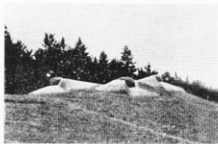
PHOTO NO. 11.—The three-turreted work is here seen from the enemy side. It is not yet camouflaged, the towers and masses of concrete show up strongly against the dark background. The turrets are so deeply embedded in the concrete that it is only just possible to fire out of the loopholes.
