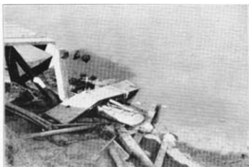
4.—Float and decking of Japanese assault bridge.
