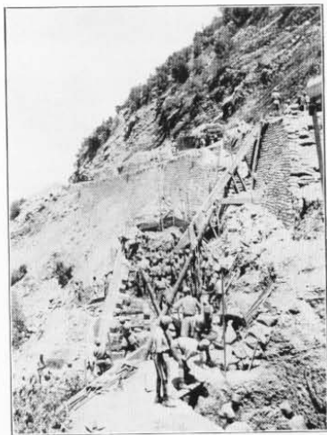
8.—Razani retaining wall. Temporary repair is above.
