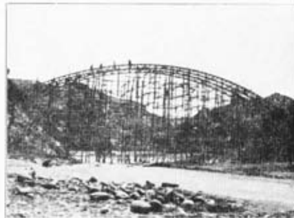
7.—The steelwork of the arch ribs completed.
