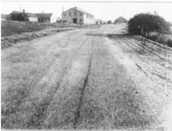
3.—The surface after partial rolling.
