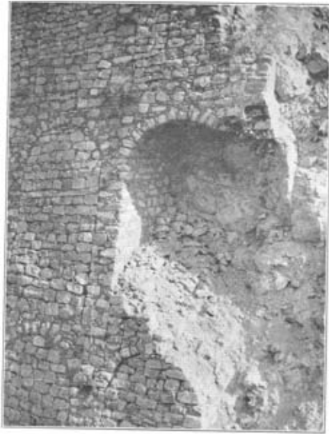
3.—The unsupported counterfort arch.
