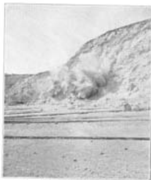
5.—Firing a batch of charges.
