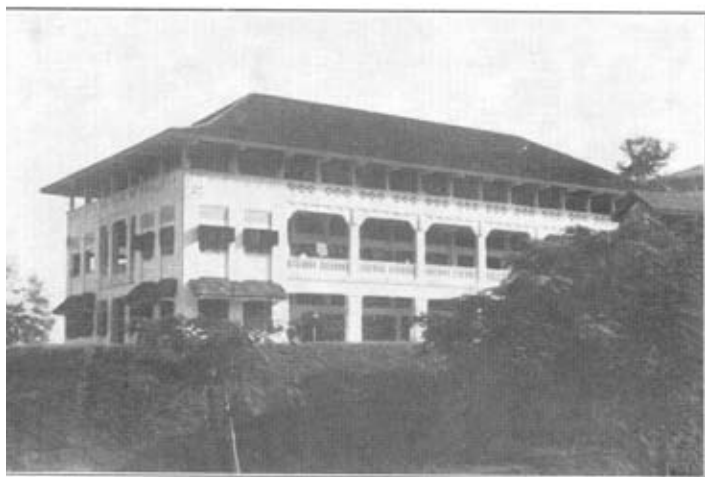
Barrack block with pitched roof: windows of offices, etc., on ground floor provided with protective overhanging canopies.
