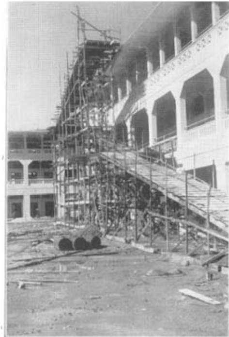
Scaffolding showing normal means of access to roof (during construction.
