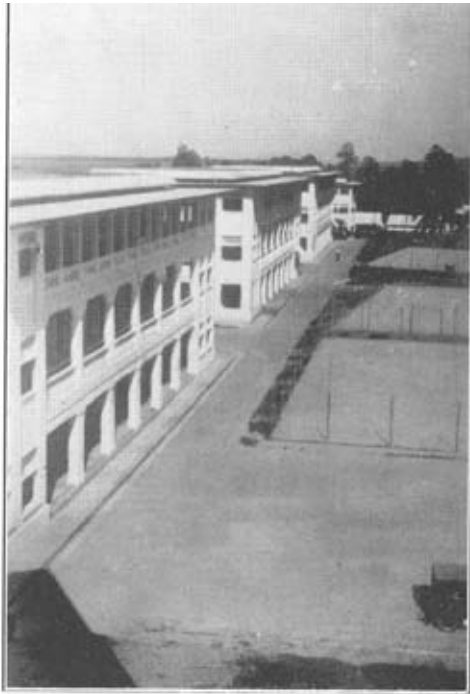
Flat-roofed barrack blocks: note high and low-level roofs separated by a clerestory grill protected by an overhanging slab.
