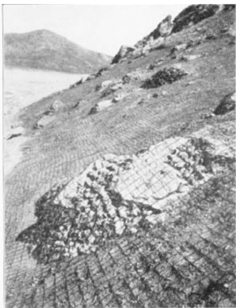
4.—Mesh pegged to the ground.
