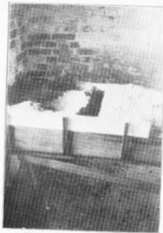
Fig. 6.—Trench Revetments.
