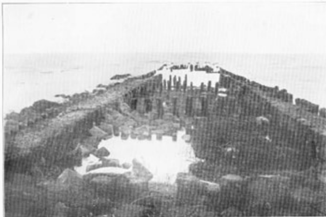
19.—Storm damage, Groyne No. 4, Borkum. This groyne has since been demolished. 1931
