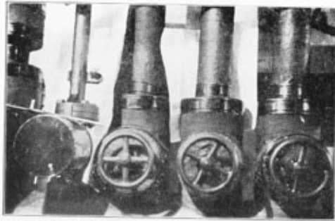
Fig. 6.—Valve insulation, as made and fitted by Cairo Water Co.
