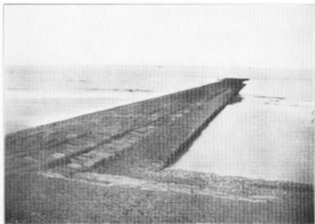
17.—Groyne, D.1. Norderney. Sides supported by iron retaining wall. 1931.
