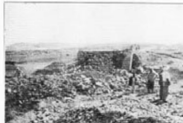
4.—View of demolished bridge from north west, showing how the abutment wing wall have been forced outwards at top.
