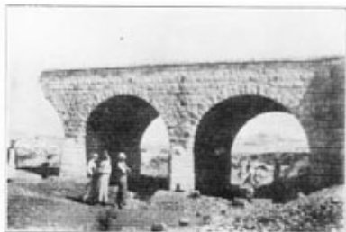
1.—View of bridge from south-west. Pier charges laid. Sappers placing weep-hole charges. P.W.D. coolies looking on.
