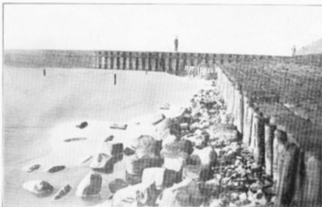
20.—Erosion near the junction of Groyne No. 7 and the protected outer dune, Borkum. June, 1934.
