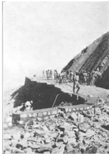
Photo 8.—Approach nearing completion, retaining wall completed.
