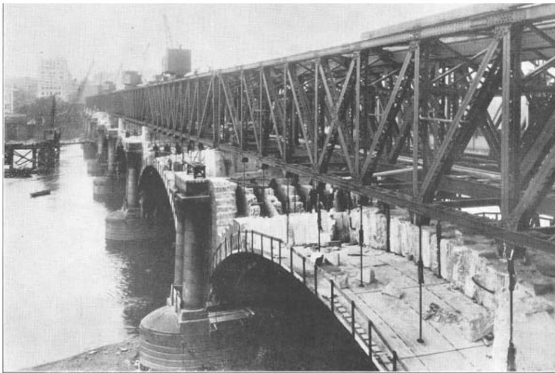
Fig. 6.—Arches partly reduced to 12-foot wide "middle strip."
