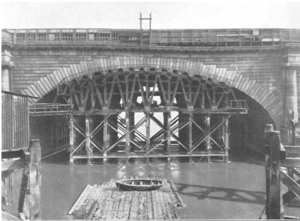
Fig. 3.—Arch No. 5 supported by piling.
