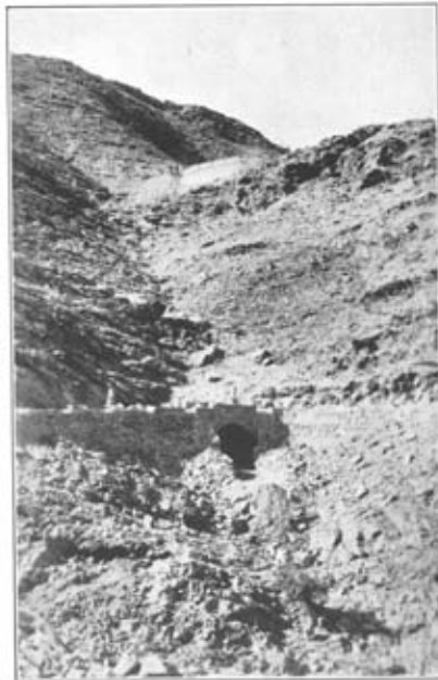
Photo 4.—A culvert constructed of 8ft-span elephant-shelter sections, with masonry abutments, and 1st loop at top.
