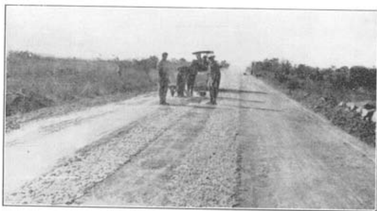
Photo 2.—Spraying and rolling strips.
