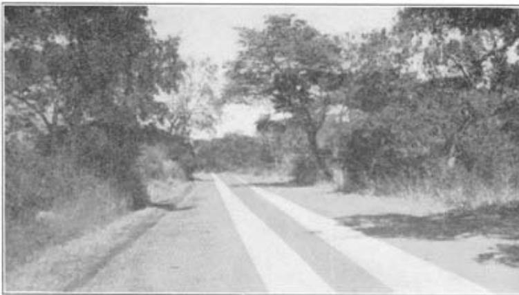
Photo 4.—Concrete strips near Salisbury, S. Rhodesia.
