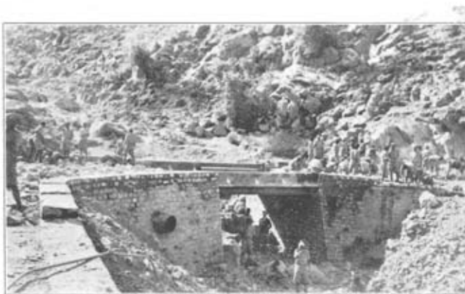
Photo 9.—15-ft. R.C. slab bridge on girders nearing completion.
