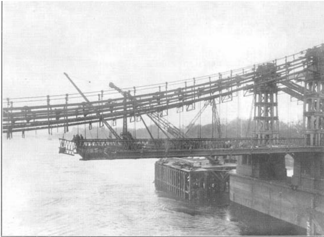
3.—Dismantling steel deck and hangers of old bridge. Temporary suspension bridge in position giving access to chains.
