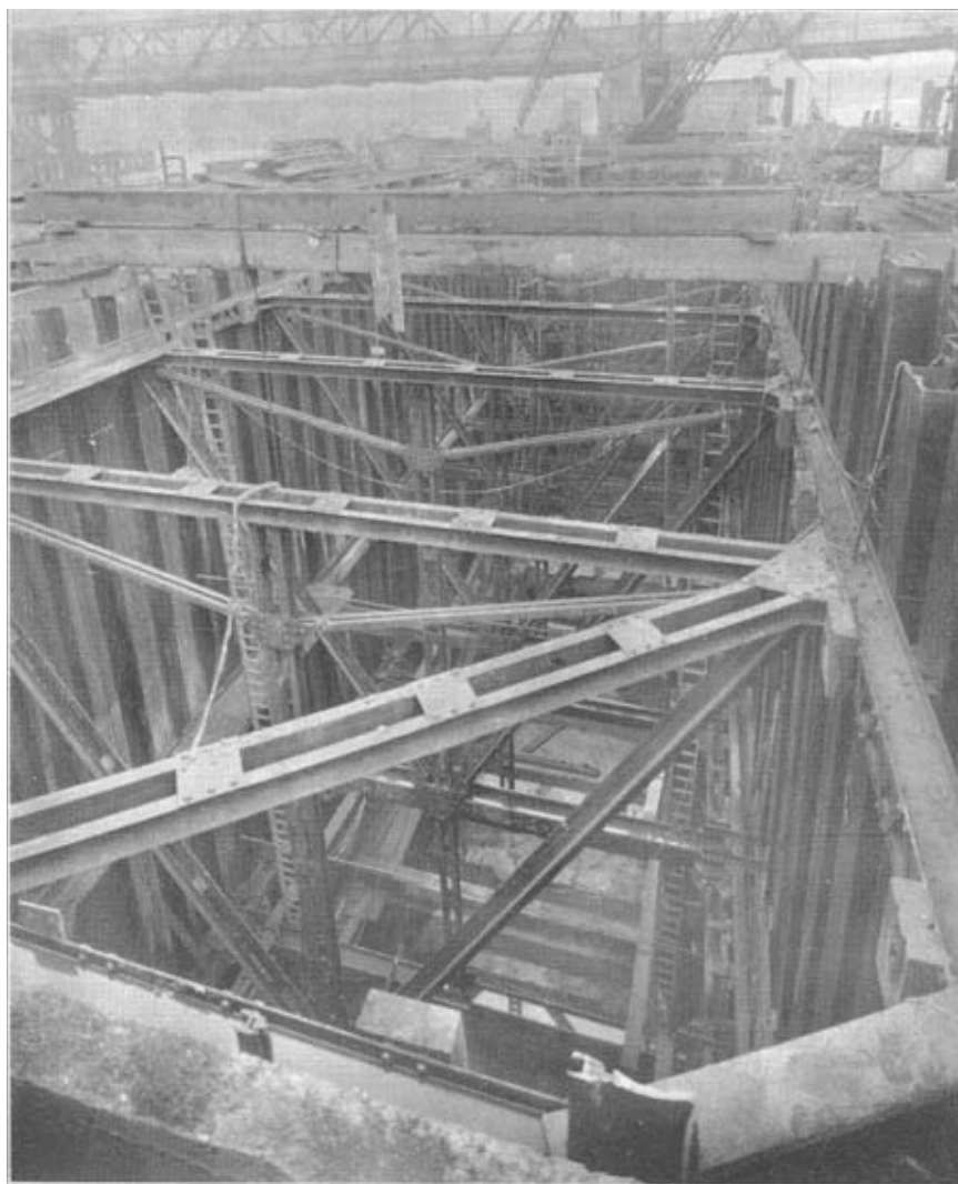
6.—Looking down into cofferdam, showing new foundation 58 feet below high water
