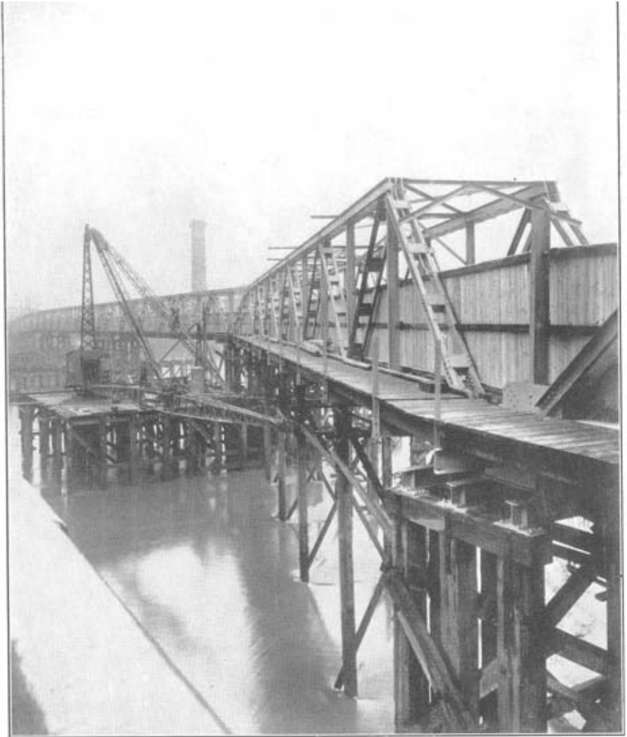
2.—Temporary footbridge nearing completion, showing contractor's gangway.
