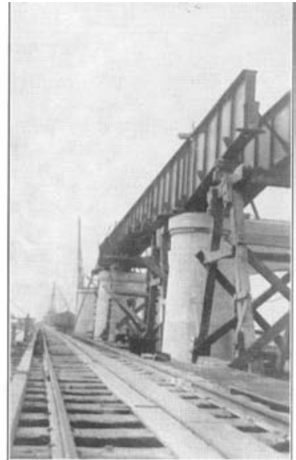
The first pair of girders (55 tons) ready for rolling into position on piers.
