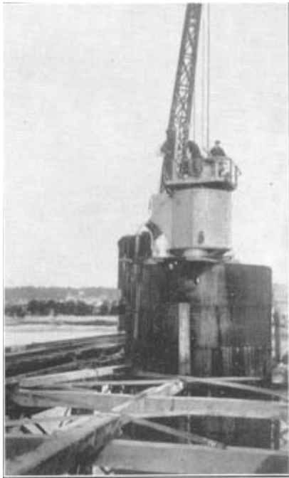
Air lock at top of compressed air caisson. North side piers.
