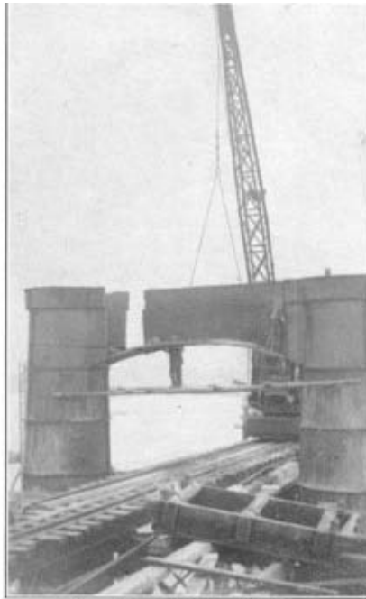
Assembling steel pier shuttering.
