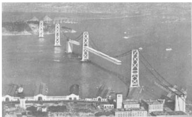
6.—San Francisco-Oakland Bridge during construction.
