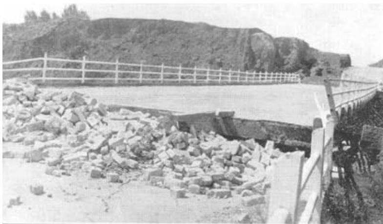
Baleli Bridge. Subsidence of abutments.
