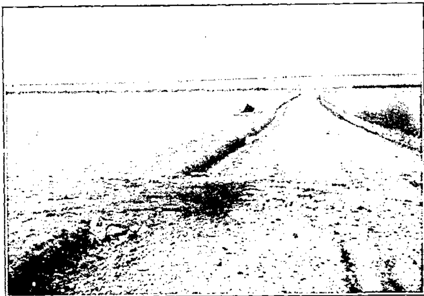
The Terolas surface after 1 year showing untreated side entrance.
