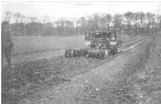
No. 5.—Mixing with disc-harrow after first application of "Terolas."
