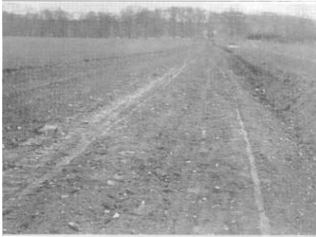
No. 1.—Graded roadway before treatment
