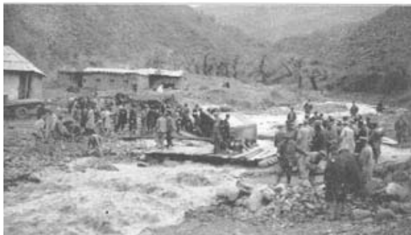
5.—Second temporary bridge across a spate; the lorry seen in the background broke the first one.
