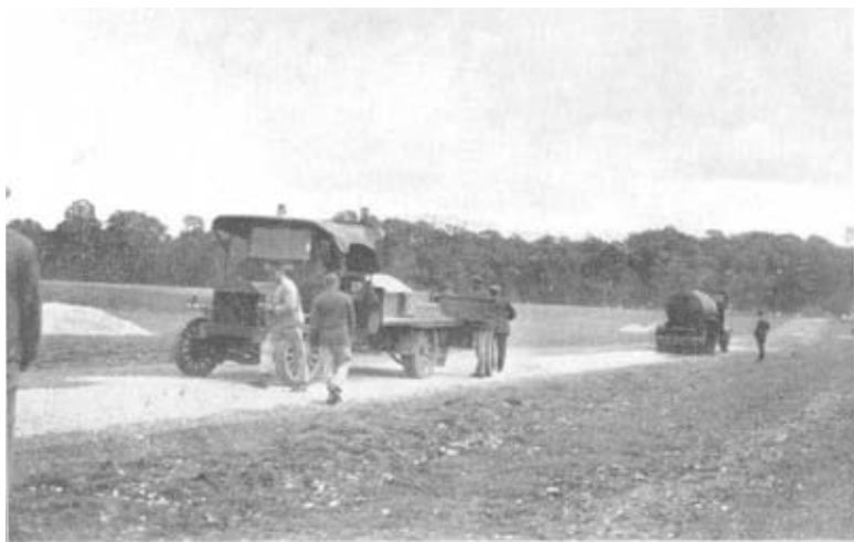
No. 6.—Appearance of road before and after surface dressing.
