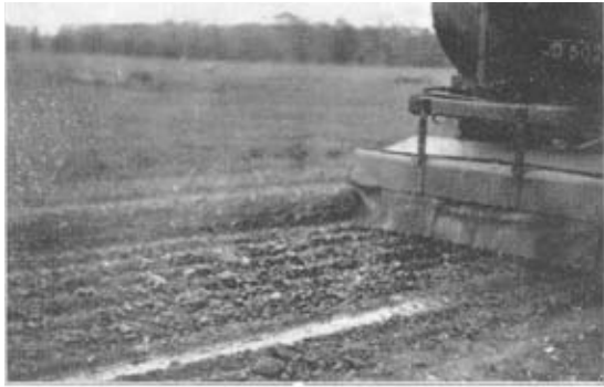
No. 3.—View of pressure tank lorry spraying "Terolas."
