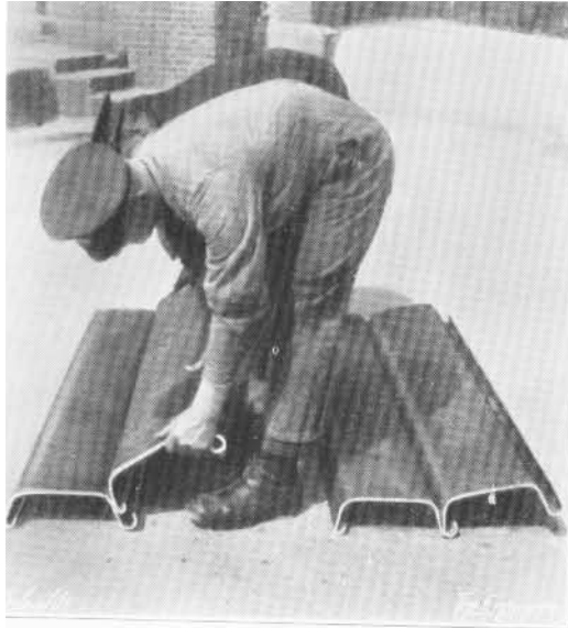
Laying the channels.
