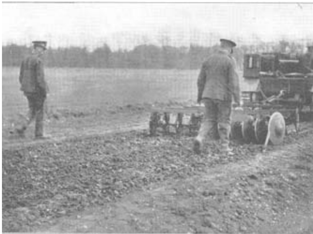
No. 2.—Disc-Harrow preparing surface for treatment.
