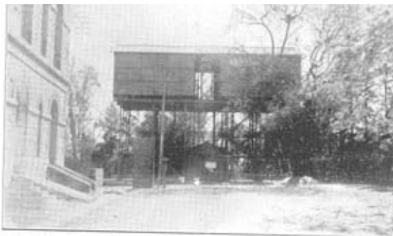
Photo 5.—Reservoirs with chlorinating plant on platform between and control house under.
