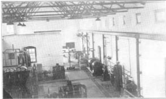
Photo 1.—Power station and workshop. Note grouped air auxiliaries on right.
