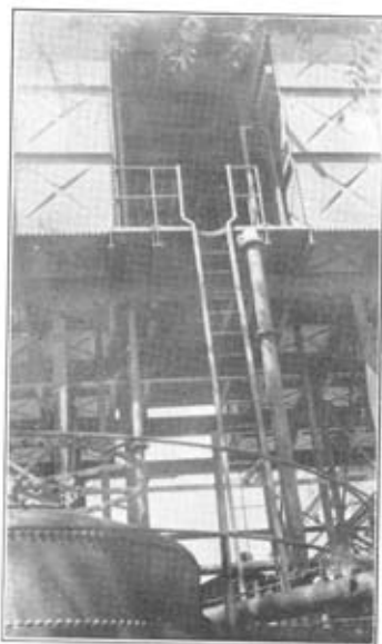
Photo 6.—Reservoirs. Note continuous roof, platform between tanks, gantry for hoisting chlorine cylinders.
