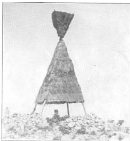
Photo 11.—Typical major triangulation beacon. Height to neck about 20 ft.; to top, 25 ft. Side at base about 12 ft.
