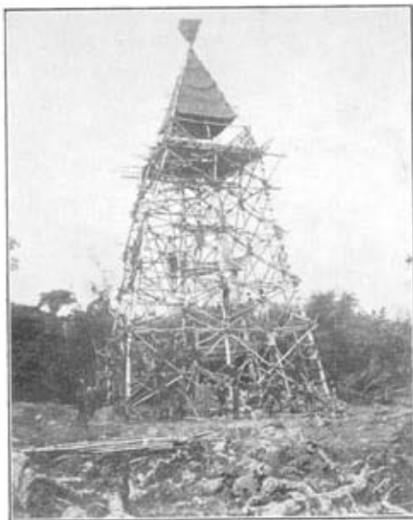
Photo 10.—Kisebwe Tower beacon, 40 ft. to platform, 62 ft. to top of beacon—Mweru-Tanganyika section.
