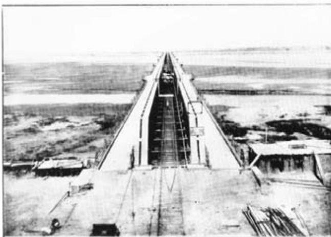
Photo. 5.—General view from the Shahpur end of the completed bridge, showing the cantilevered roadways with crossing stations.
