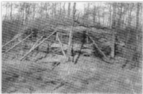
6.—Somerset House (Bn. H.Q.)—an early attempt at a built-up, bullet-proof "dug-out"; the roof was splinter and, we hoped, also weather-proof.
