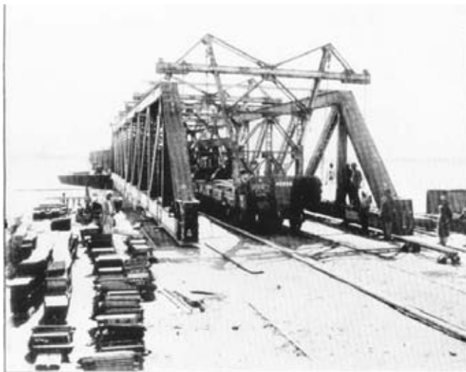
Photo 4—View showing traveller on abutment ready for moving the outer girder into position.
