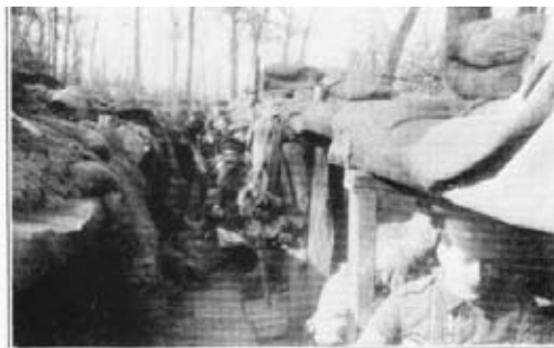
9.—The front line (actually in March, 1915)—the shallowness of the trench and inadequacy of protection in the cut and cover dugouts will be noticed.
