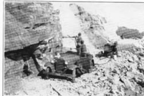
4.—Dressing the face by means of several shallow bore-holes
