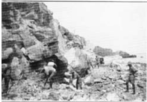
3.—Clearing after firing a simultaneous line of charges.
