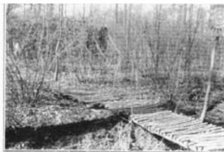
5.—PLOEGSTEERT WOOD.—An example of our original type of corduroy path or "duck walk."
