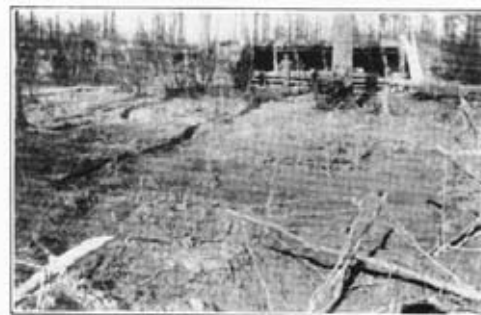
7.—Support line breastworks (splinter-proof) which were started late December or early January, '15. Note the early form of barbed wire "gooseberries" ready to be taken out at night.
