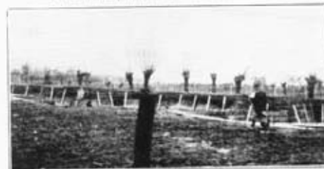
3.—The "Torres Vedras" line behind (or west of) the village—semi-breastwork type of construction.
