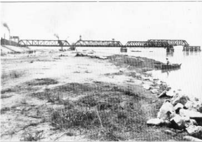
Photo 2.—Showing the inner girder of span No. 4 being launched.
