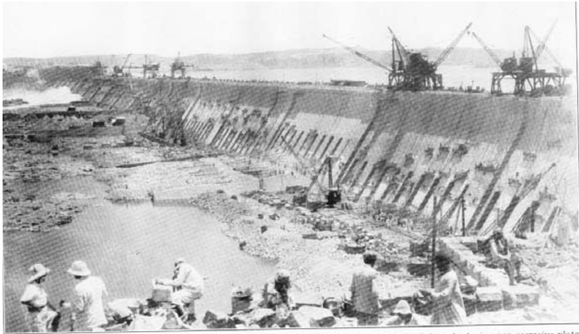
General view of the downstream side of the dam from the west end: showing dressing face of dam for laying non-corrosive plates to take the new masonry addition. The heightening of the dam is approaching from the east,
