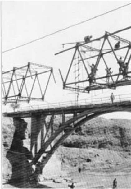
No. 5.—Lashing the jibs in position.
