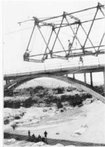
No. 6.—Preparing to detach a transom, before lowering it into the river bed.
