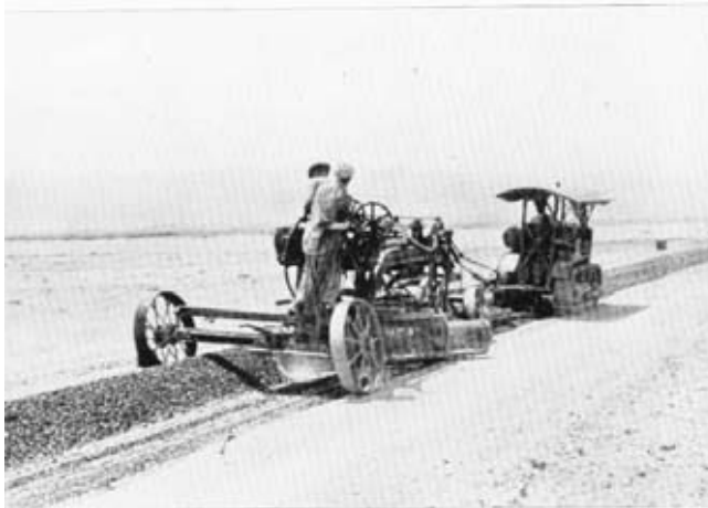
2.—Forming the windrow after the first application by tractor and grader fitted with a mixing blade.
