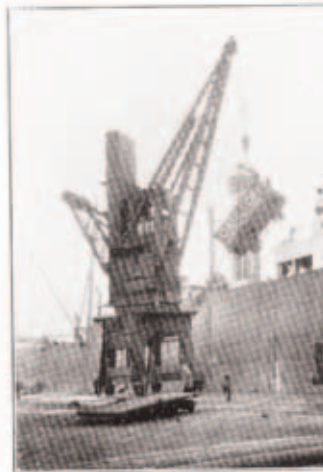
Photo 4.—Lifting 20-ton end-door wagon for unloading.
