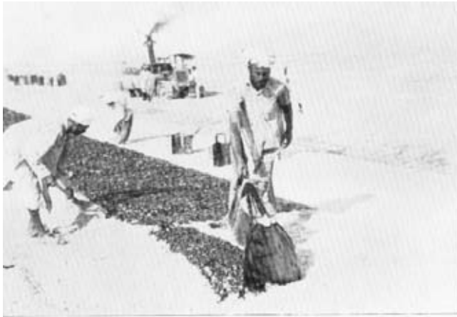
1.—Pouring the hot bitumen by hand.
