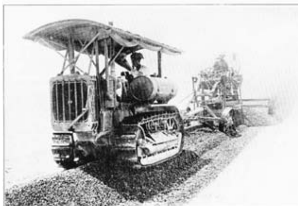
5 —Tractor and grader fitted with mixing blade carrying out the final mixing operations.
