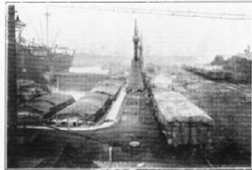
Photo 6.—Bad railway lay-out for jetty.
