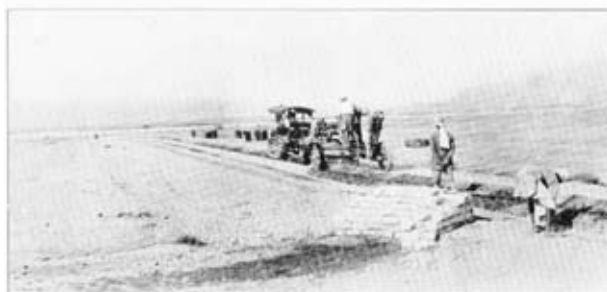
3 and 4.—Moving the windrow across the road to ensure all particles being coated with bitumen.
