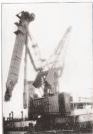
Photo 1.—4-ton lifting jib electric crane, fitted with bucket elevator.
