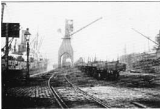
Photo 7.—Good railway lay-out for jetty.
