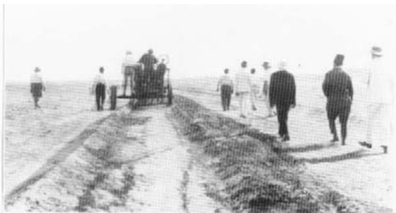
First blading, after first application of the asphalt.
