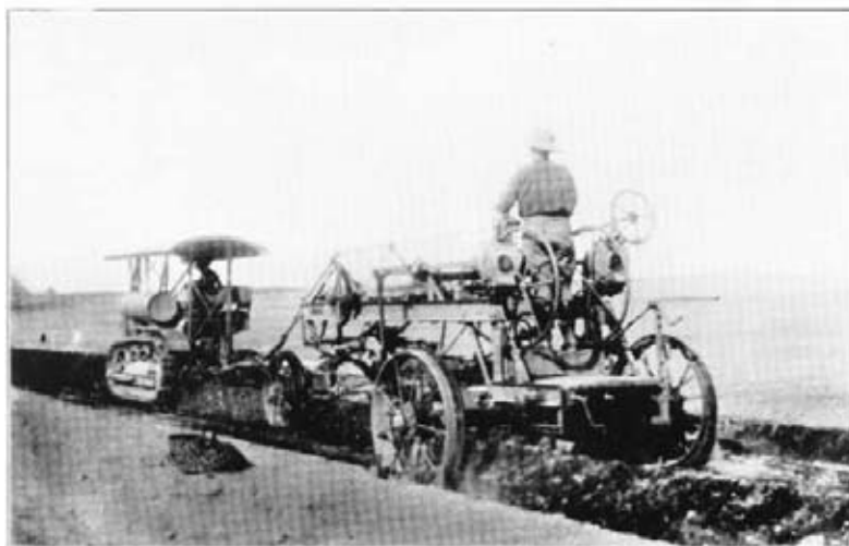
Final blading, preparatory to spreading of mix.
