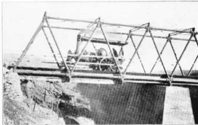
Photo 9.—View of subsidiary span, showing concrete counter-weight in end two bays.
