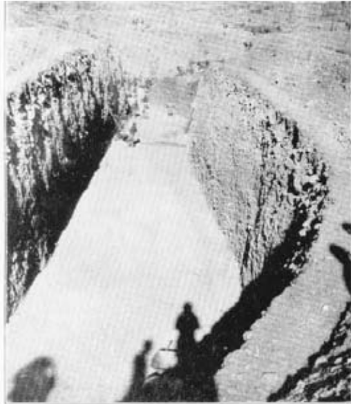
Photo 8.—View of left bank cutting completed.
