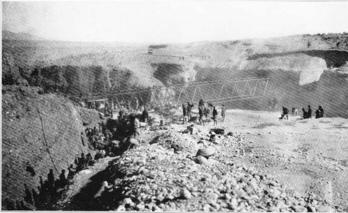
Photo 7.—Showing excavation of approaches, and launching in progress.
