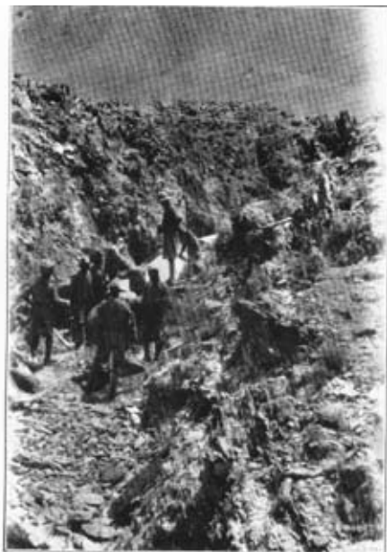
Photo 3.—Laying "armco" culvert in concrete in side nullahs at mile 21 \frac{1}{2} .
