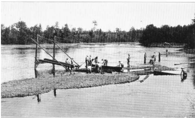
4 —Pier and approach under construction. Flying bridge.
