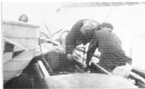
2.—Drilling the spinnaker boom for the fid.
