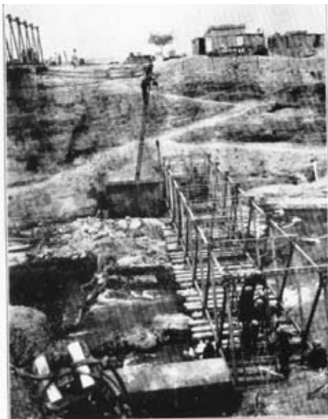
Photo No. 3.—Showing the Inglis Bridge on its temporary platform and the piers on to which it is to be hoisted.
