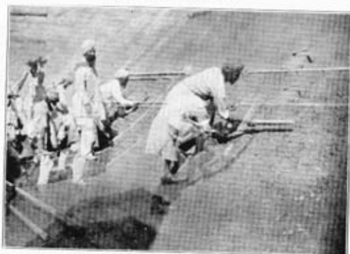
9.—Plastering Side Wall.
