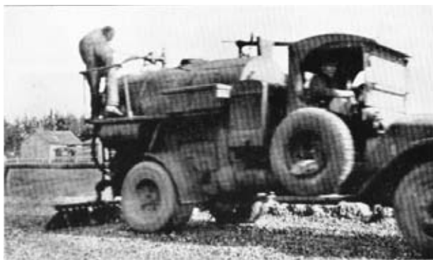
No. 1.—The application of the emulsion by means of a pressure distributor.
