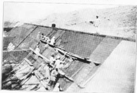
8.—Plastering Side Wall.
