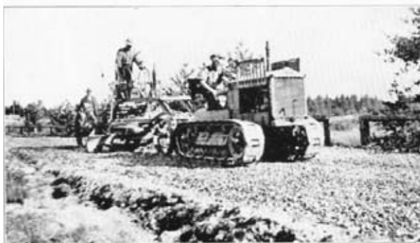
No. 2.—A tractor-drawn grader in operation.
