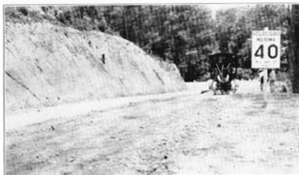
No. 3.—A grader forming a windrow of scarified material.
