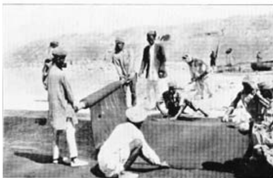
6.—Laying the Cotton Membrane.
