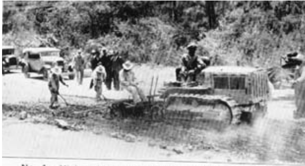
No. 4.—Mixing with a tractor-drawn disc harrow and spike drag.
