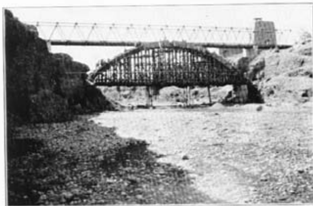
Photo No. 4.—Showing how the contractor was able to support his centering on the temporary Inglis, well clear of another spane.
