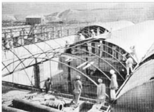
11.—Laying Roof Sheetting.
