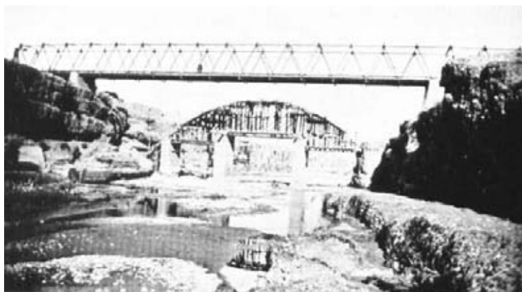
Photo No. 1.—Showing the old Inglis Bridge and the false-work for the new R.C. Arch Bridge.
