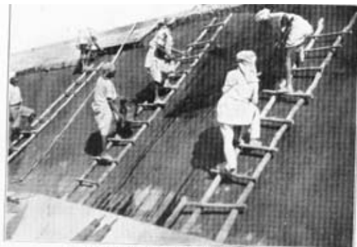
7.—Applying "Flintcote" Work on Corners.
