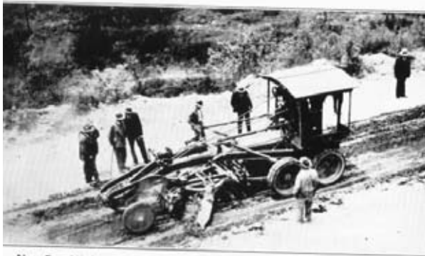
No. 5.—Mixing with a self-propelled grader controlled by one man.
