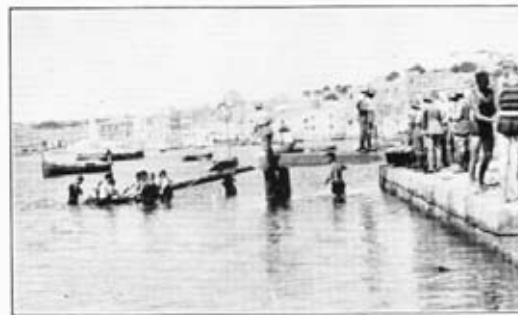
Photo 4.—During construction; note distance-piece men. Trestle about to be raised, chess-laying proceeding.
