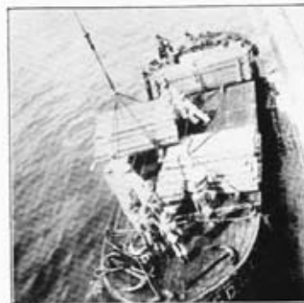
Photo 8.—Loading pierhead lighter from a warship. Note deck marked to show where packages are to rest and bearers under each package.
