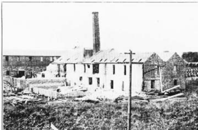
Photo 8. —Immediately after firing charge; note difference in height of chimney
