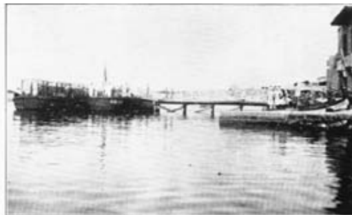
Photo 2.—Pier with lighter loaded with horses in horse boxes alongside. Pier built from pierhead lighter to shore.
