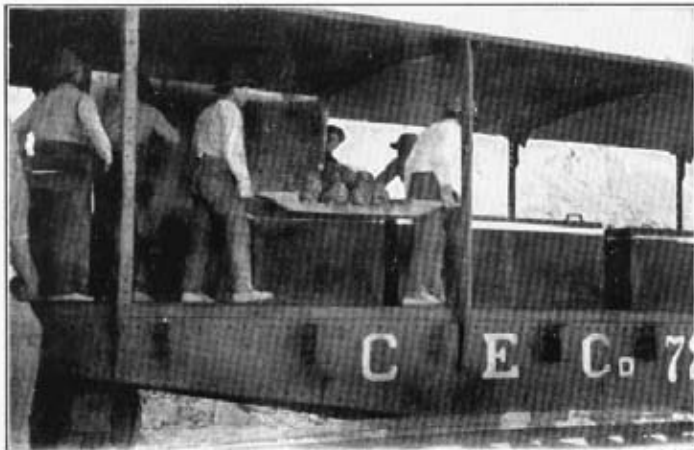
Photo No. 4.—Unloading of L O X cartridges from the soaking boxes at the site of the blast.
