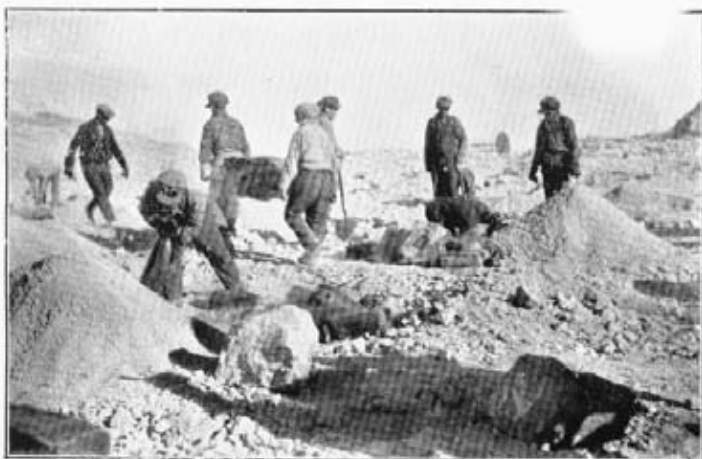
Photo No. 2.—Charging bore holes with L.O.X.
