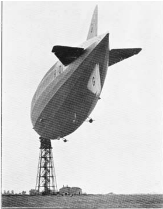
FIG. 10.—A STERN VIEW OF THE R 101.—Note the fins and rudder and elevating planes. Also the "Power Eggs" and the control cabin. Each portion of the rudder is 45 feet high.
