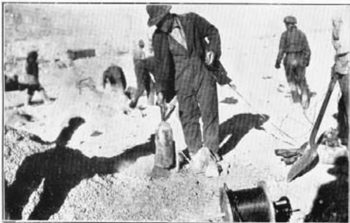
Photo No. 1.—Dropping 32 lb. L.O.X. cartridge down bore hole.
