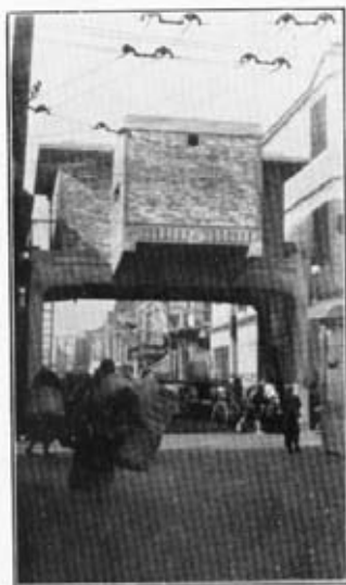
Photo (d).—Blockhouse "E," just beyond the cross-roads of two narrow streets. It is raised on a framework of reinforced concrete, and the caponier gives facilities for firing up and down the street at right angles to the one in the photo.
