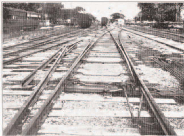
Photo of Saidpur Yard, showing Metre-Gauge skewed to one side.
