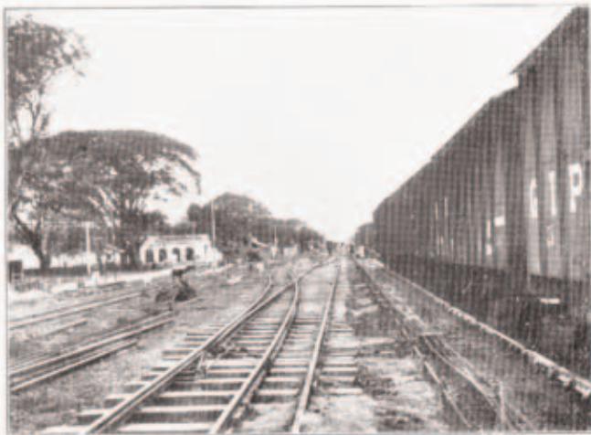
Saidpur Yard, showing termination of three-rail track.
