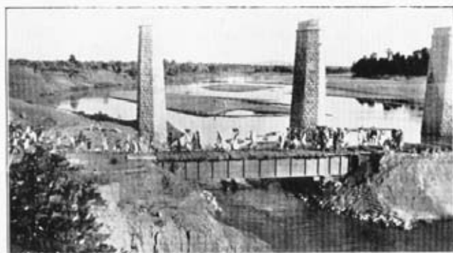
The 40 ft. span in position,
