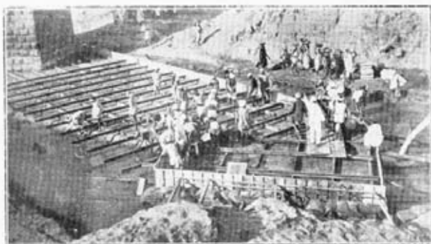
The reinforcing rails in position and further concreting in progress.
