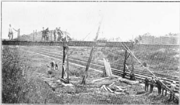
3.—Lowering a girder into position.
