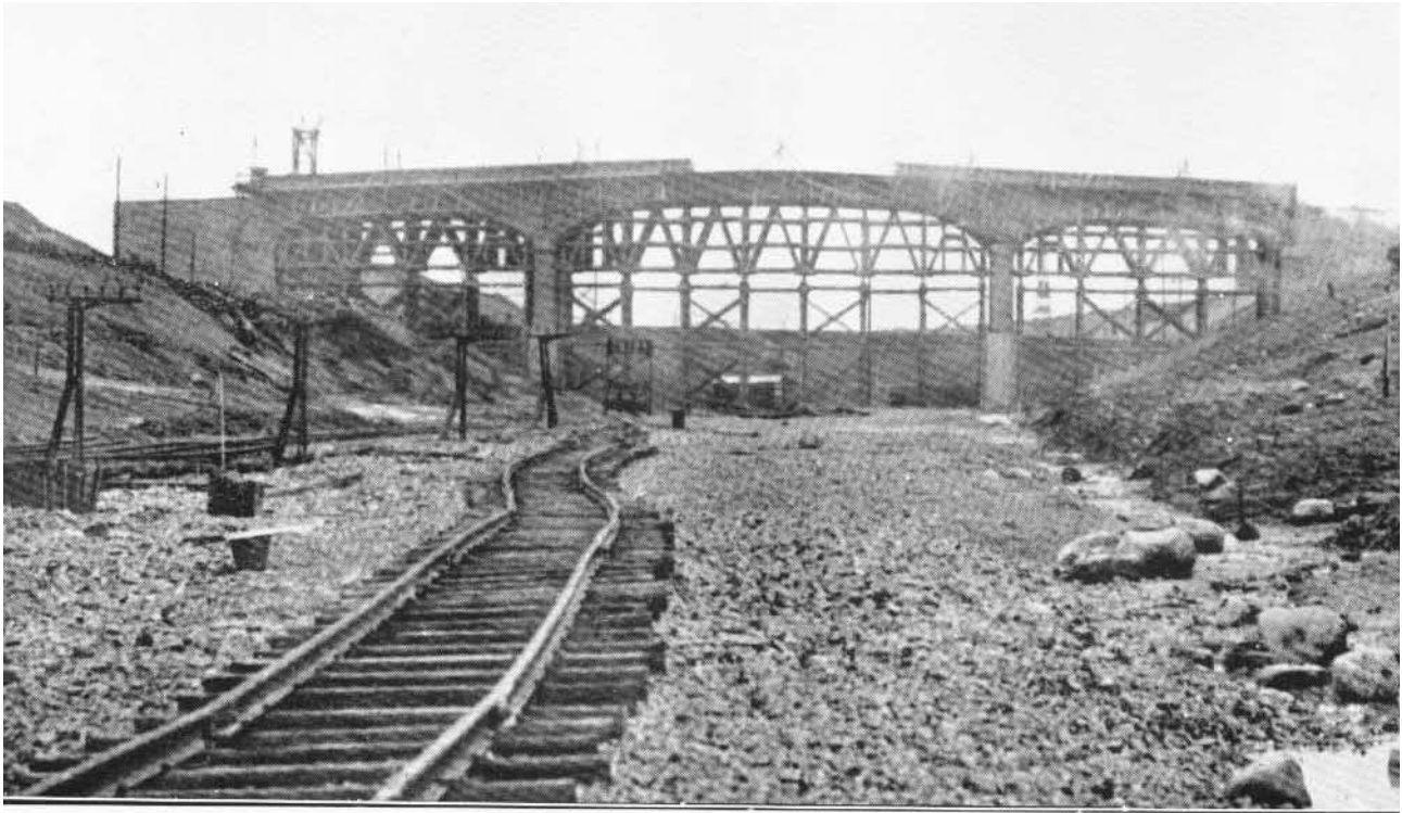
Photo 3.—Reinforced Concrete Road Bridge under construction.
