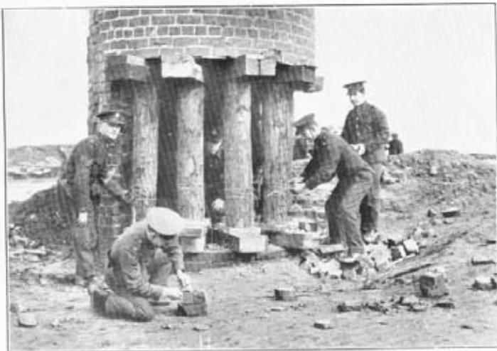
No. 1. View showing arrangement of sills, wedges, props, caps, and packing pieces.
