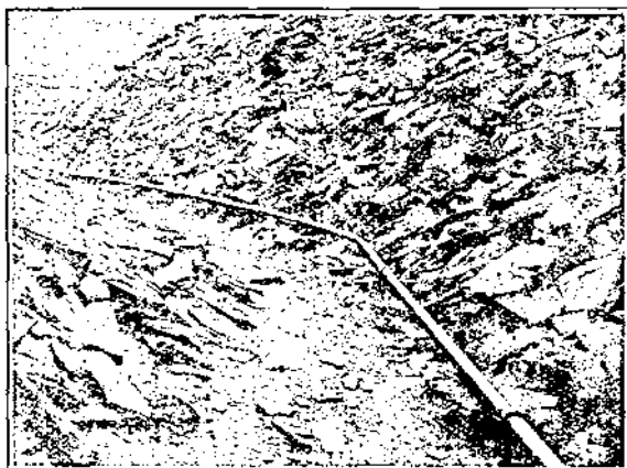
Victaulic Compressed Air Line at the Moel Faen Slate Quarries.
