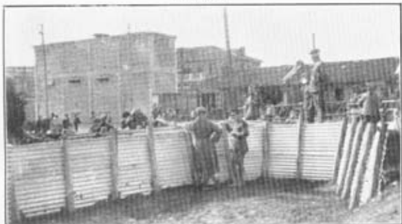
No. 1.—C.G.I. revetment with earth filling completed to give all-round fire. Type used in No. 1 sector.
