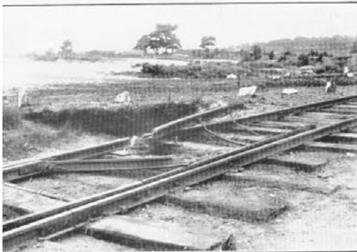
60-LB. RAIL.—Six slabs gun-cotton at the crossing.
