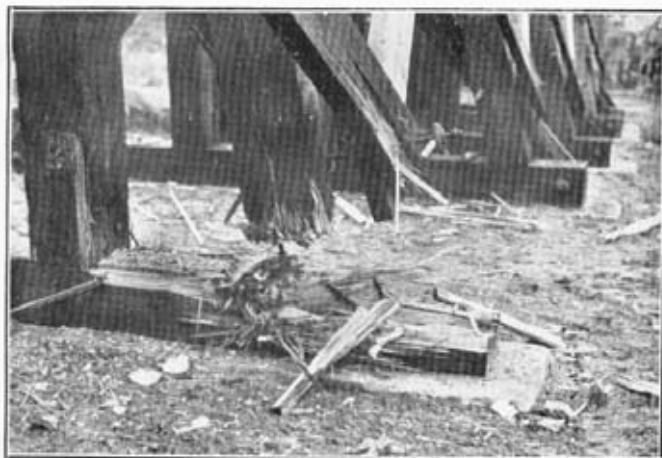
DAMAGE TO THE SINGLE TRESTLE.—Right-hand, raker and bottom sill damaged. Left-hand, raker and both verticals undamaged.
