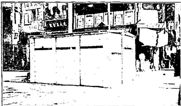
No. 12.—Concrete blockhouses: loopholes cut as required for M.G. and L.G. 4 ft. \times 1 ft. \times 4 in. slabs with double X.P.M. reinforcement. Erection, 12 men from 6 to 8 hours: digging holes for posts, additional 3 to 9 hours, dependent on quality of road; a pneumatic drill was sometimes available for this and for making holes for entanglement pickets.
