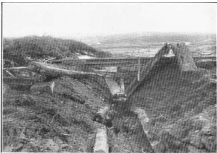
The effect of two 5-lb. charges of gun-cotton in a culvert in a 2-ft. bank. Only one charge exploded.
