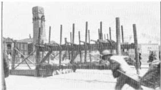
No. 10.—Shows method of mounting large gates on crown of bridge where excavation into roadway was not permitted.
