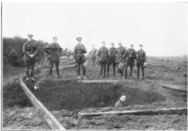
NO. 1 CRATER.—29-lb. ammonal. Diameter, 28 ft. Depth, 7 ft. Craters Nos. 2, 3 and 4 are in background.
