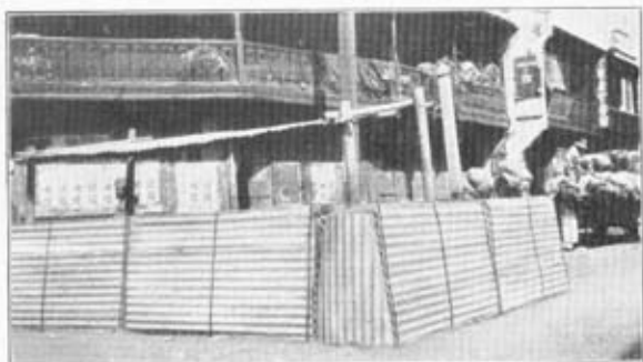
No. 2.—C.G.I. boxes with \frac{3}{4} in. \times \frac{1}{8} in. flat iron bands around and internal ties, to hold sand. Used by Italians to replace sandbag posts when the latter had deteriorated.
