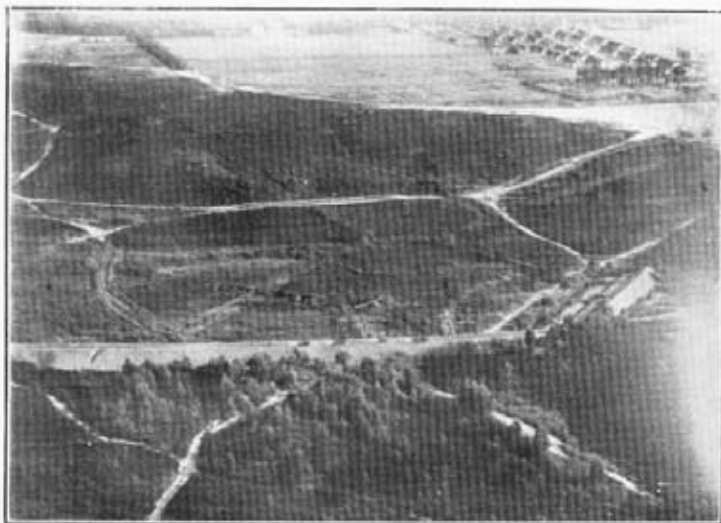
AEROPLANE PHOTOGRAPH OF MINE CRATERS.—No. 1 (ammonal) is on the right. No. 5 (to the left) misfired. In the background, the enemy camp at Longmoor. The embankment is 12 ft. high.
