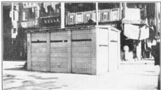
No. 12.—Concrete blockhouses; loopholes cut as required for M.G. and L.G. 4 ft. \times 1 ft. \times 4 in. slabs with double X.P.M. reinforcement. Erection, 12 men from 6 to 8 hours; digging holes for posts, additional 3 to 6 hours, dependent on quality of road; a pneumatic drill was sometimes available for this and for making holes for entanglement pickets.
