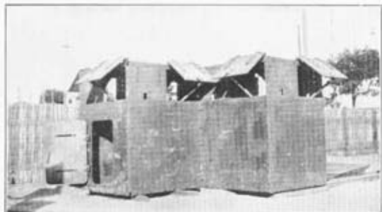
No. 11.—Experimental M.S. blockhouse. Sufficient parts were ordered to make (a) two 10 ft. \times 3 ft. blockhouses, (b) one 10 ft. \times 10 ft., (c) one L-shaped 10-ft. frontage as in picture. Made in 5 ft. panels, two thicknesses of 3/8 in. M.S. sheets being used. Loop-hole plates 3/4 in. M.S. hinged for coolness in summer. Roof angle 3/8 in. M.S. Erection of 10 ft. \times 3 ft., seven men 4 1/2 hours.
