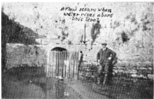
Experimental Strainer of old fencing standards across inner end of culvert. 5 ft. x 4 ft.
