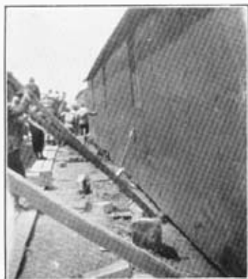
Levers in position for raising.
