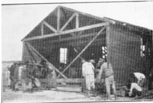
Cross-strutted ready for moving.
