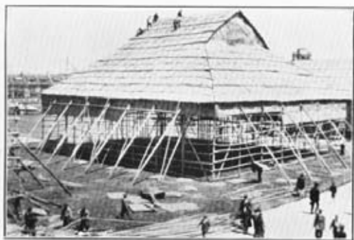
Thatched hangar under construction.
