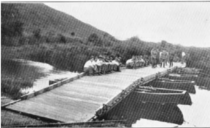
Pontoon Bridge completed.
