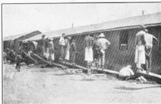
Raising by "walking the plank."
