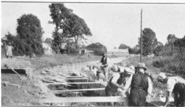
The Bend at Rock Terrace.—Fixing Shuttering.
