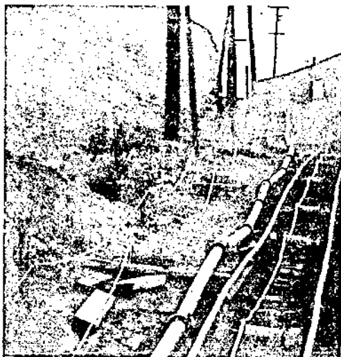
The illustration shows a 21" bore Victaulic line which was rapidly laid at night for an emergency at a colliery, by workmen who had never seen a Victaulic joint before.
