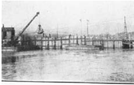
PHOTO. 1. Cofferdam at the Weir.
