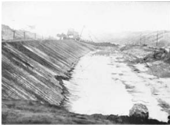
PHOTO. 3. Head Canal under Construction.
