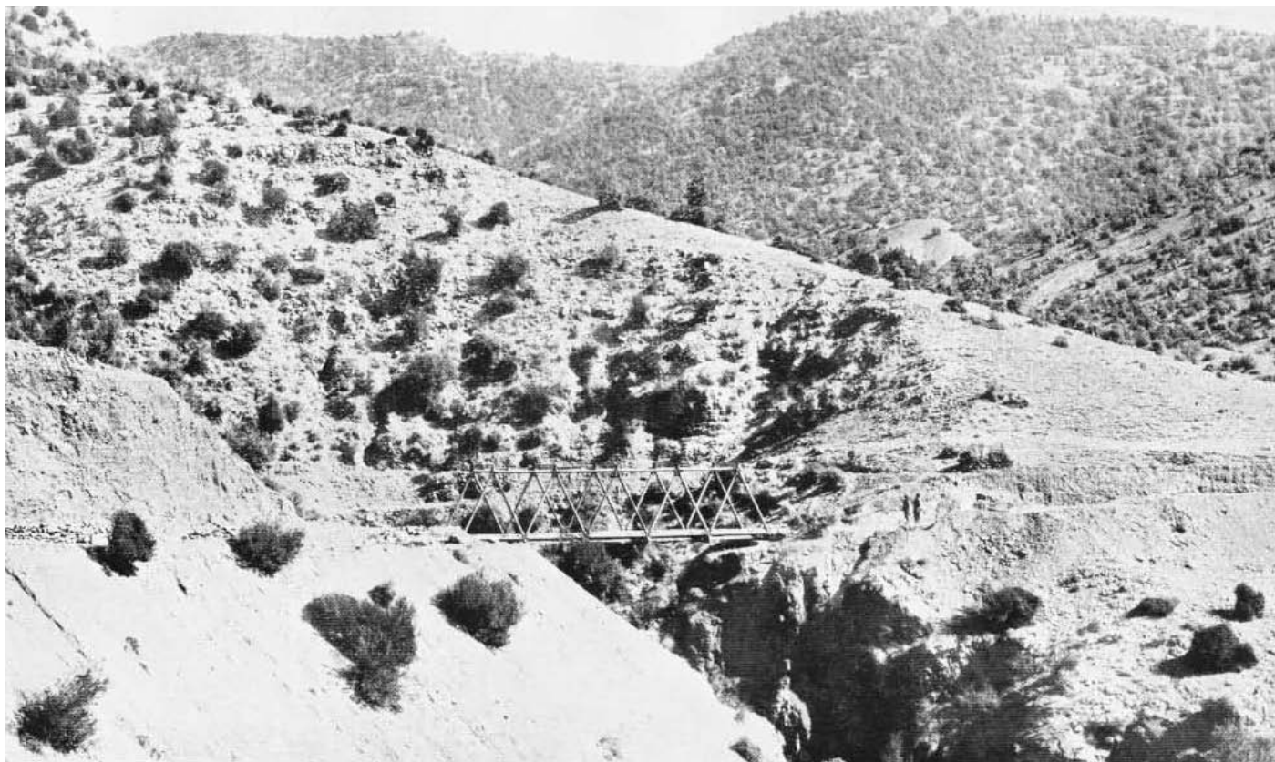
The Erection of an Inglis Bridge in Waziristan
