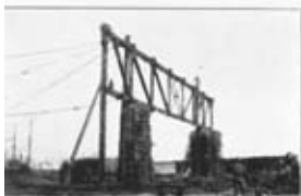
Photo 6.—100-ft. Girder in position ("H" Hangar).
