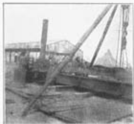
Photo 5.—Straightening a bent column with improvised oven.
