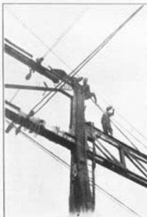
Photo 7.—Bolting in 100-ft. Girder ("F" Hangar).
