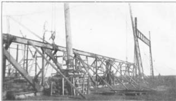
Photo 4.—100-ft. Girder assembled and ready for erection ("F" Hangar).
