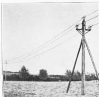
FIG. 6.—German 45,000-volt Line and Anchor Pole: Stranded Aluminium Line 120 sq. mm.
