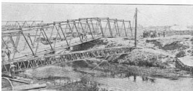
4, 5, and 6.—Box Girder Bridge. Launching 96' girder.
