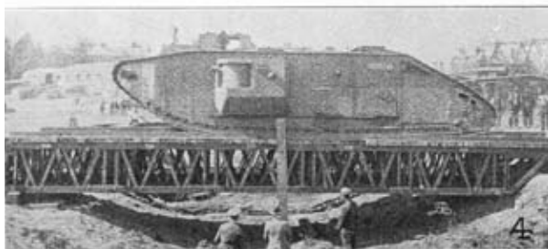
3.—Box Girder Bridge. 48' long—3-girder Bridge. 35-ton Tank on bridge.
