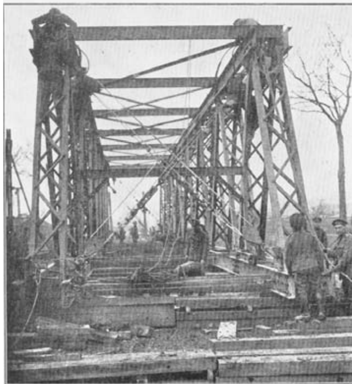
Photograph II.—Launching Hopkins 120 Ft. Type Span. View from near bank, showing temporary wire rope cross bracing.
