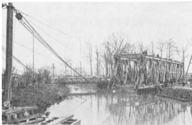
Photograph III.—Launching Hopkins 120-Ft. Type Span. Span launched 45 ft. Fixing slings for main launching tackle.
