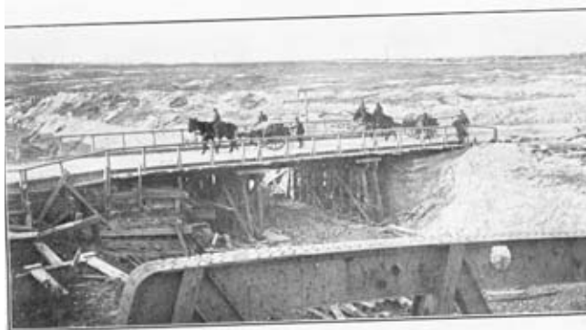
Photograph XXXII.—Canal du Nord : R.S.J. Spans for all loads.
