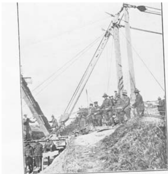
Photograph XXXI.—Havrincourt, Canal du Nord : Attachment of the tackle to the heads of derricks.
