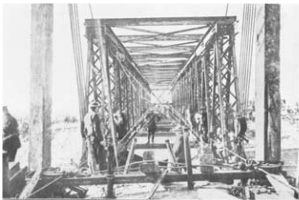
Photograph XXVIII.—Temporary Diagonal Wire-rope Bracing.
