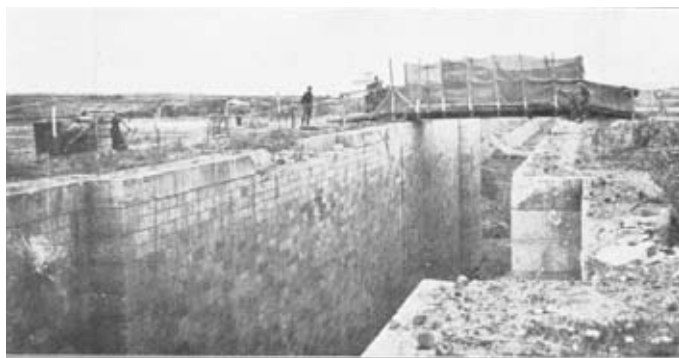
Photograph XXXIII.—Canal du Nord. Typical R.S.J. Span across Lock.
