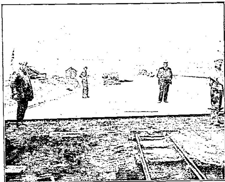
EXMOUTH SEA DEFENCE WORKS. Expanded Steel-Concrete Slope and Roadway. Length One Mile; Total Width of Roadway, 65 Feet. Mr. SAMUEL HUTTON, U.D.C. Engineer and Surveyor.
