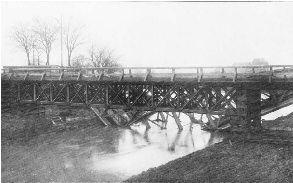
Bridge 124 \frac{1}{2} ft. span built by a detachment of ——— Field Co., R.E. Clear span of main girders, 65 ft.
