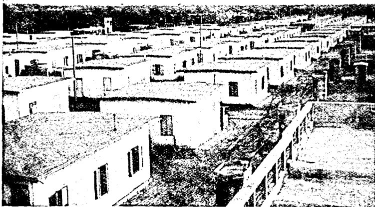
FIRE AND EARTHQUAKE-PROOF BUILDINGS AT MESSINA. Timber Stud Framing and Expanded Metal Lathing and Cement-Mortar Hollow External and Internal Walling.
