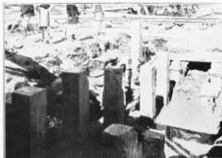
Pile heads after completion of driving.
