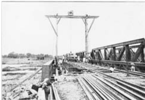
Erecting the new girders on staging carried by the old ones. New bottom booms and cross girders almost complete.
