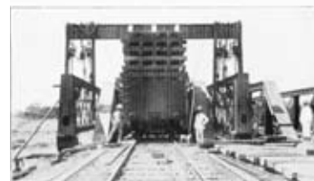
Old girders right up ready for floating.
