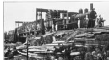
Ready to move the first span of old girders.
