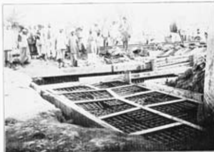
Reinforcement for slab over pile heads at abutment ready for concreting.
