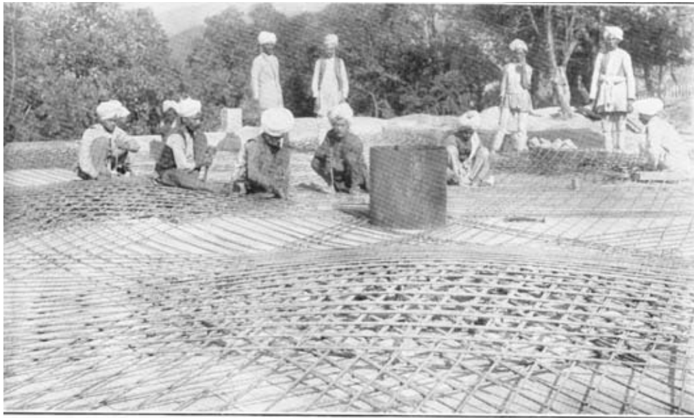
CONSTRUCTION OF A REINFORCED CONCRETE FLOOR, DALHOUSIE BAKERY.
