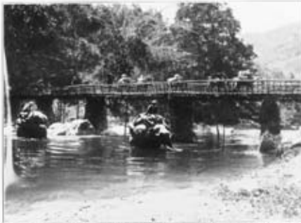
Photo 4. A good specimen of Kachin Guni Suspension Bridge (Span about 100', height of Piers over 17').
