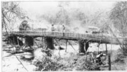
Photo 5. Kachin Guni Suspension Bridge, with intermediate trestles.
