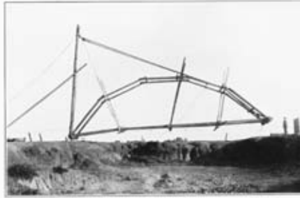
Photo 3. Swinging Complete - outer Shore Trestle over Far Bank.
