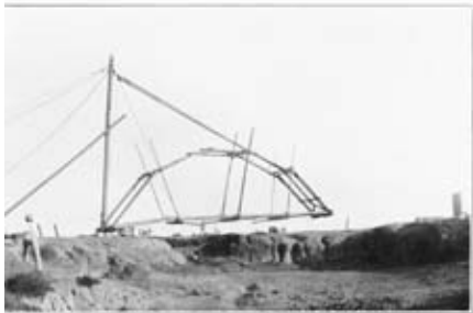
Photo 2. Swinging in progress - Bridge half-way round.
