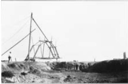
Photo 1. Bridge put together on Near Bank and outer end extended, preparatory to swinging.
