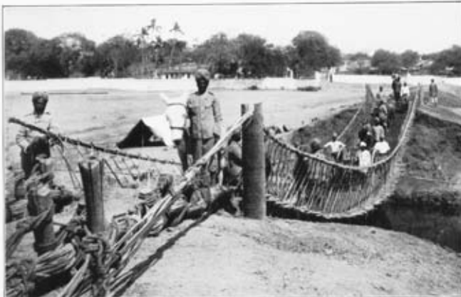
Bridge with Handrails and Windguys fixed carrying Mules and Cart to show system of Handrails, etc.
