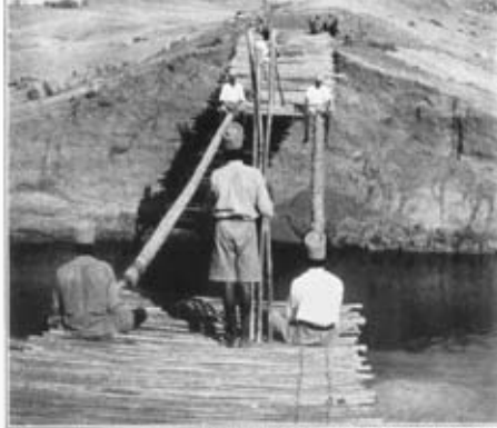
Bridge under construction showing Cables and Corduroy Roadway.
