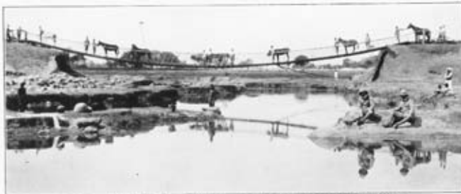
Bridge with Handrails and Windguys fixed carrying Mules and a Cart.
