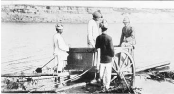
3.—RAFTS OF RUSHES. —Bullock cart (weight, 1,350 lbs.) being ferried on 5 bundles of rushes.
