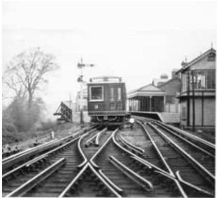
Metropolitan District Railway—Showing Third and Fourth Rail Construction.
