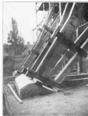
Detail of Shoring to E. Wall of N. Transept.
