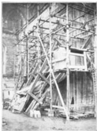
Shoring to E. Wall of N. Transept. The lower planks cover the excavations for Underpinning. B. of Water at Bottom of Excavations.
