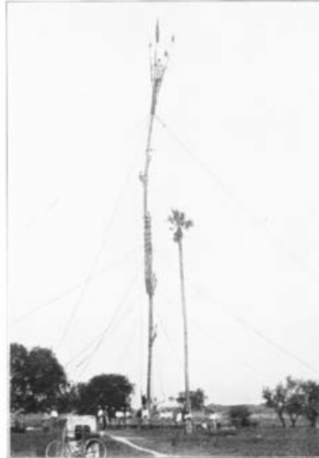
FURTHER EXPERIMENTS WITH PALM TREES AS BRIDGING MATERIAL.
