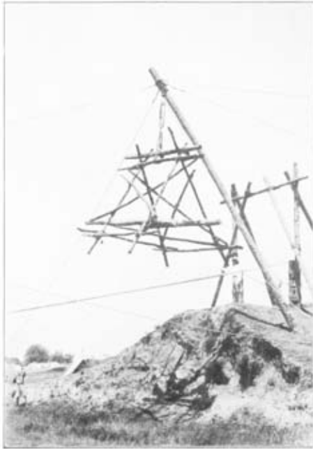
FURTHER EXPERIMENTS WITH PALM TREES AS BRIDGING MATERIAL.
