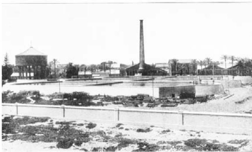
Settling Tanks and Wash-Water Tower.
